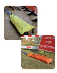
UK Power Networks are trialling new polymermembrane technology as an alternative to conventional concrete bunds at two locations
